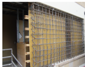
Concrete Sheer Wall
